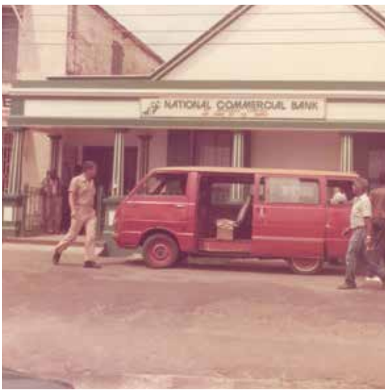
1979 The first Republic Bank Branch (then NCB), Victoria Street, Grenville
