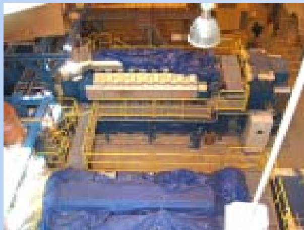
Gensets in foundations- aerial
