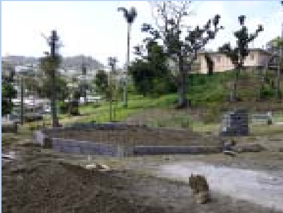
Gazebo foundation work
