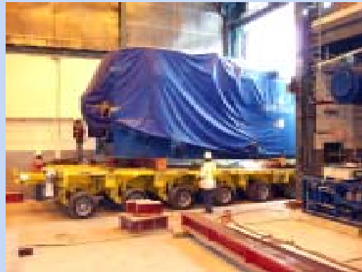
Genset being driven into place at Bruce Bain Plant
