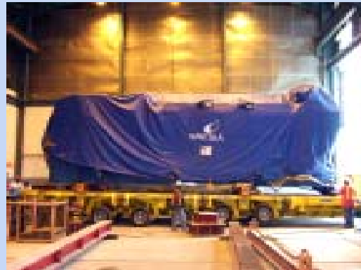
Genset being driven onto foundation
