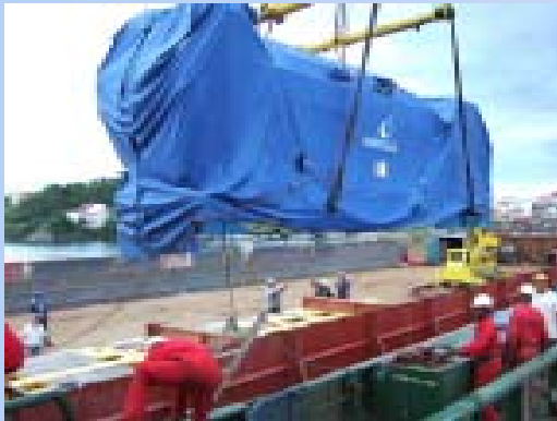
Barge for transportation to Grand Mal
