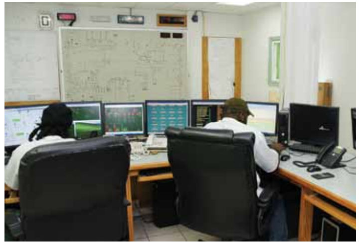
Hydro power station being monitored from Fond Cole
