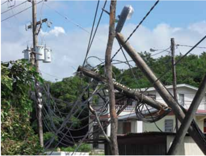
Damage to poles and lines from Tropical Storm Ophelia
