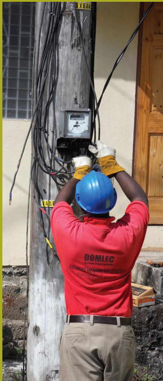
AMI installation in progress
